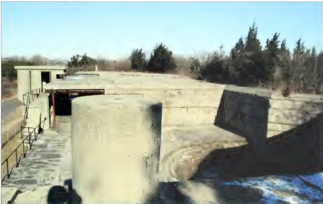
Figure 5.64. View looking north at emplacement #1 and battery commander's station, Battery Granger. Battery Granger is accessed via Hudson Drive, left, and a chain-link fence and signage have been installed between the road and battery to warn visitors of potentially hazardous conditions. Eastern red cedars, right, are heavily concentrated at the interface of the engineered slope and the battery's concrete terreplein (Olmsted Center, January 2009).
